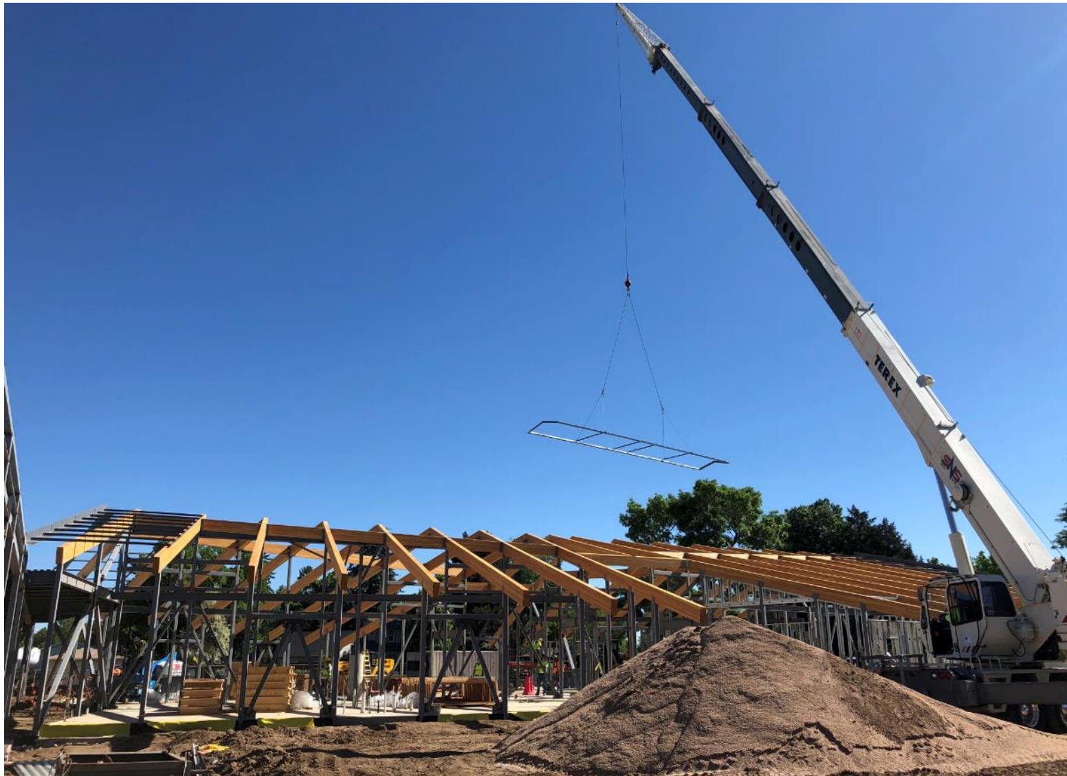
Installing steel frame for skylight.
