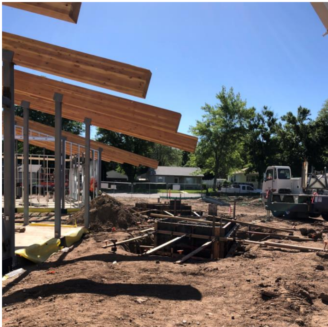
Rain chain foundations being formed.
