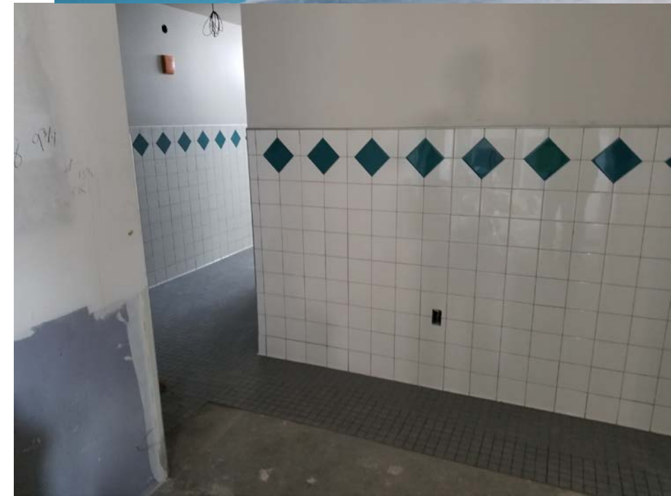
North Classroom Wing (upper level) – Restroom; Wall tile newly installed.
