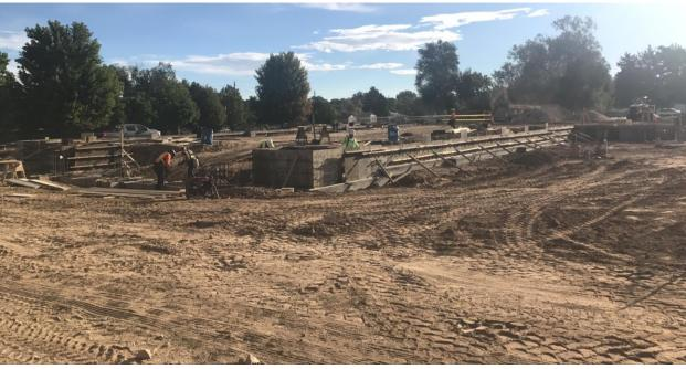
Fire Riser and Relocated Hydrant are in Place. Water Meter pit is underway.
