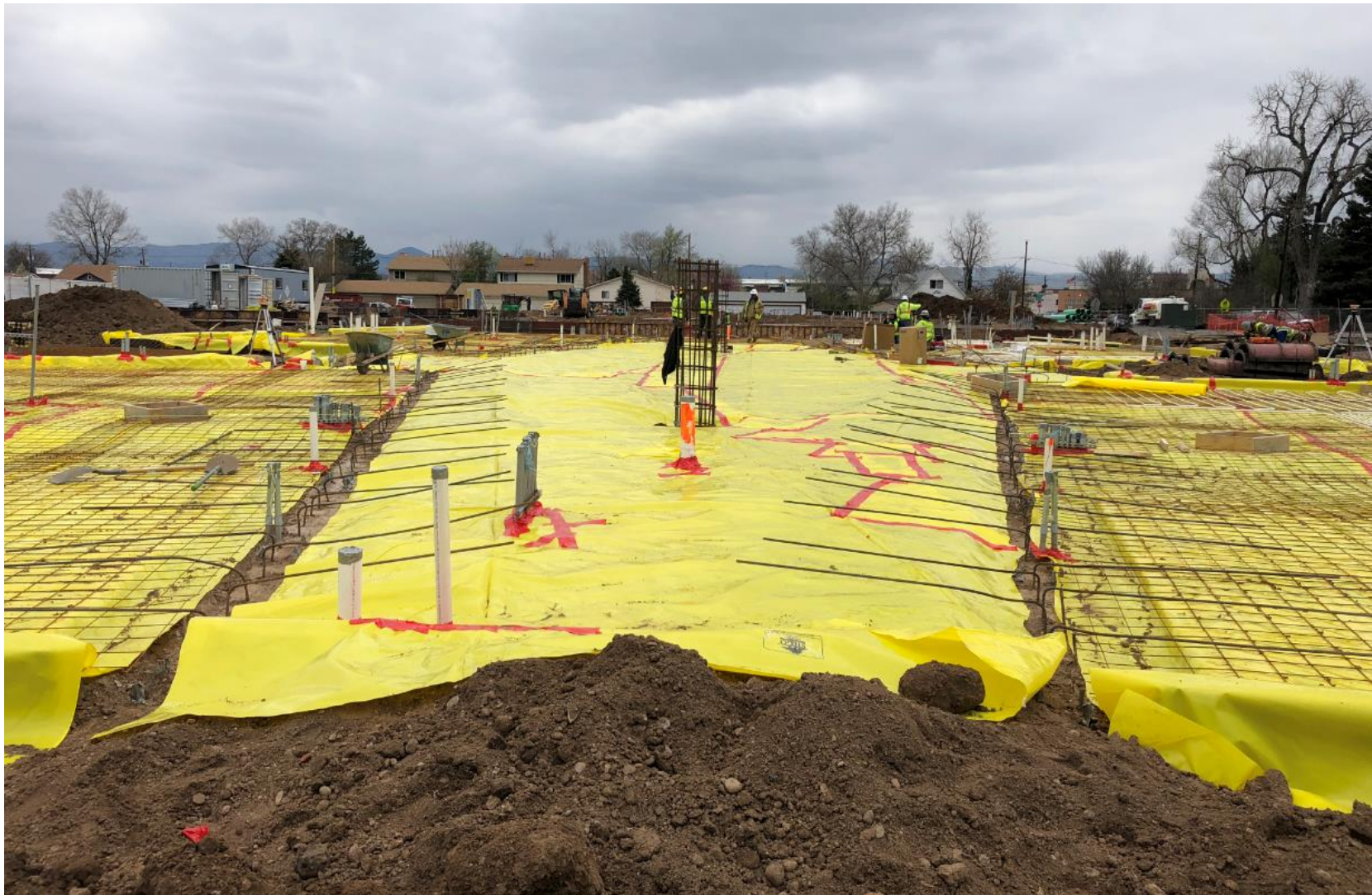
Looking West across building. Vapor barrier installed.
