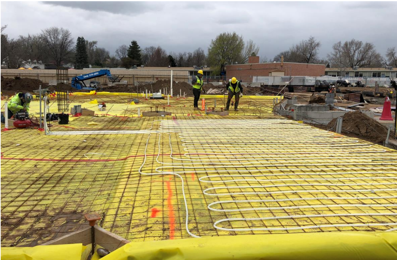
Radiant floor heating install.
