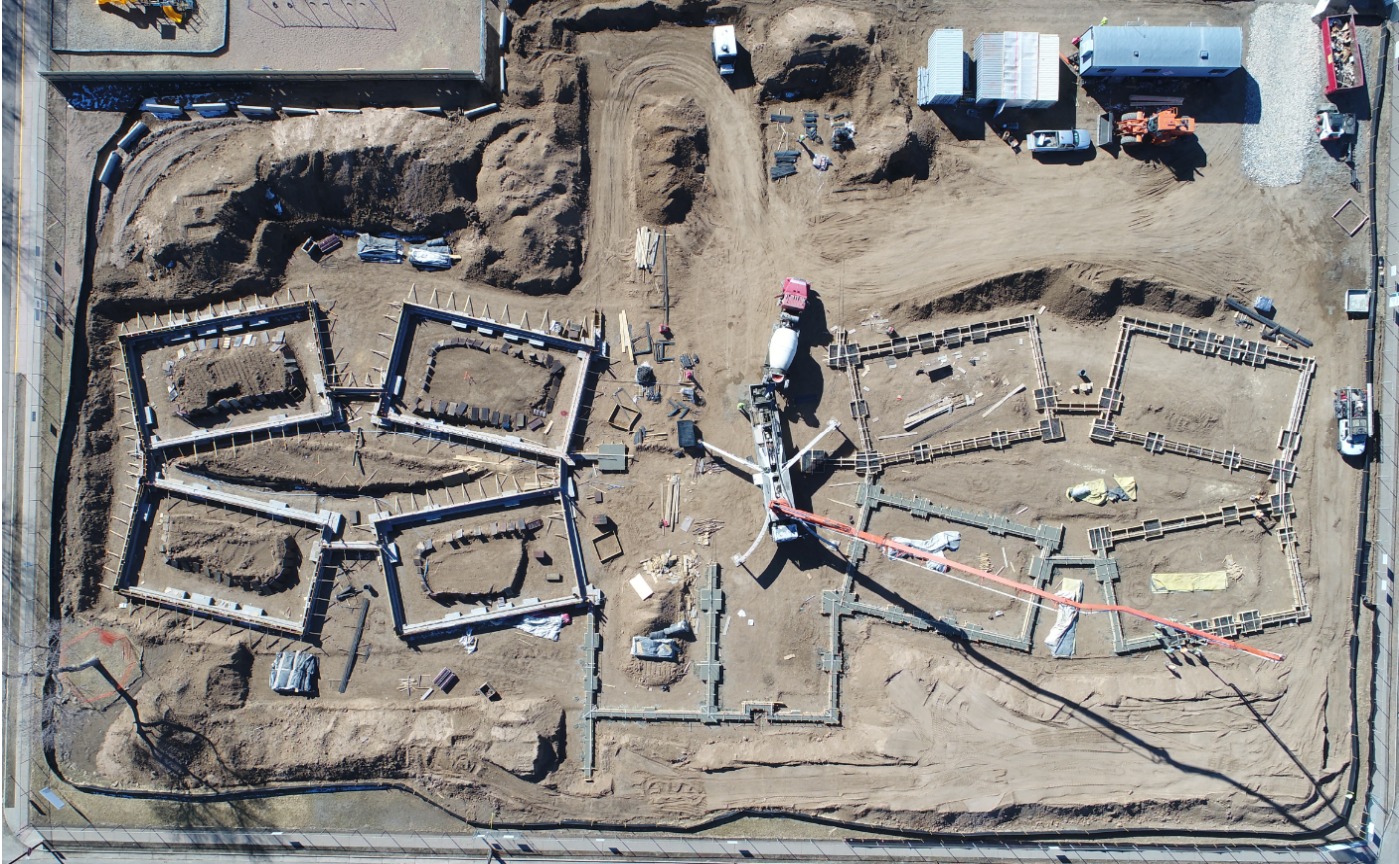
Aerial view of footings during concrete pour.
