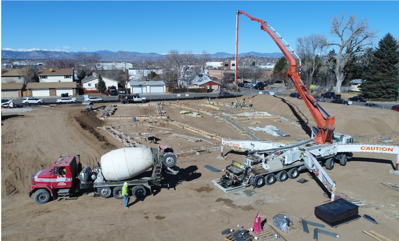
Concrete pour on West wing footings.
