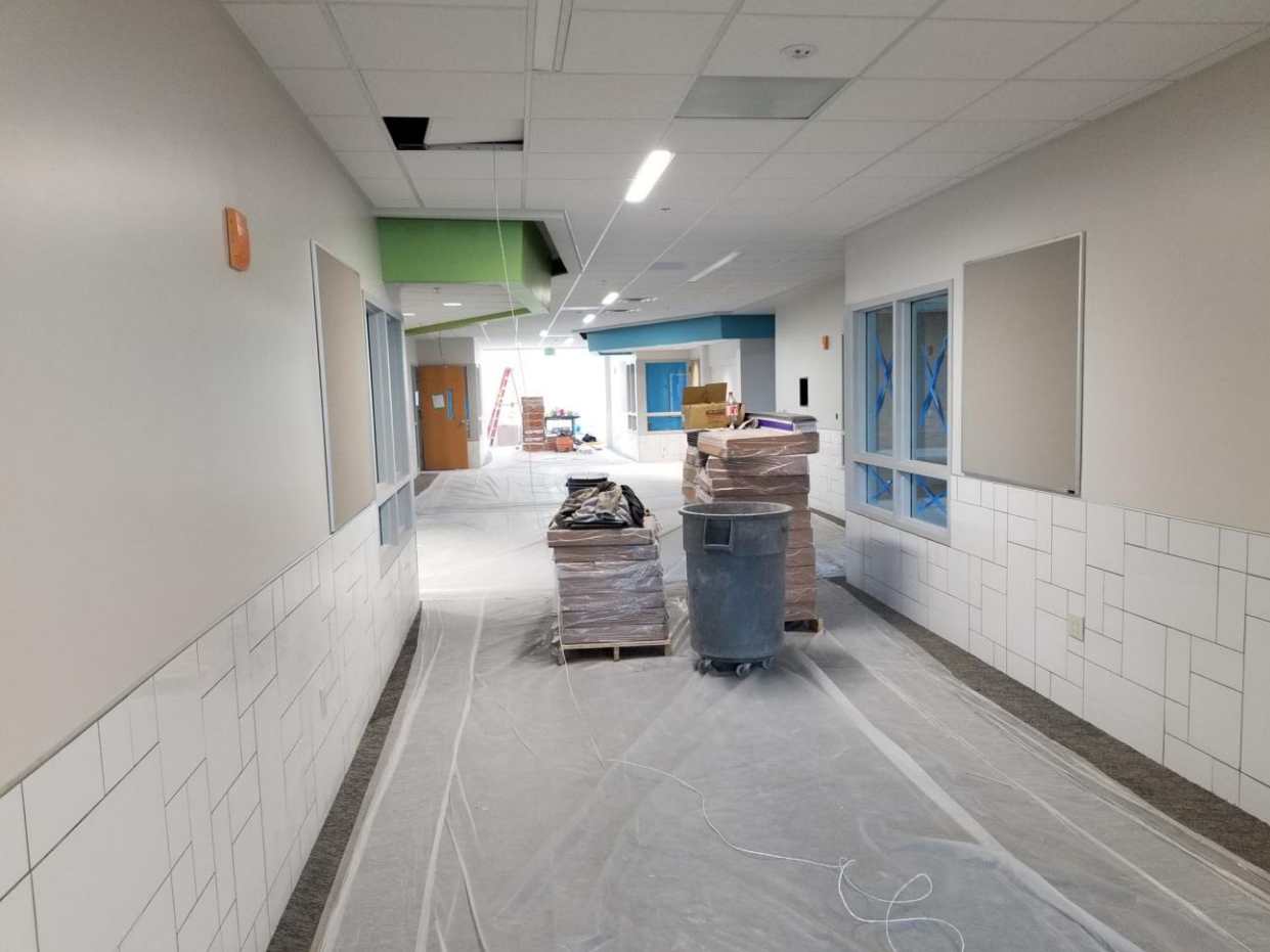
North Classroom Wing (upper level) – Tack and white boards newly installed.
