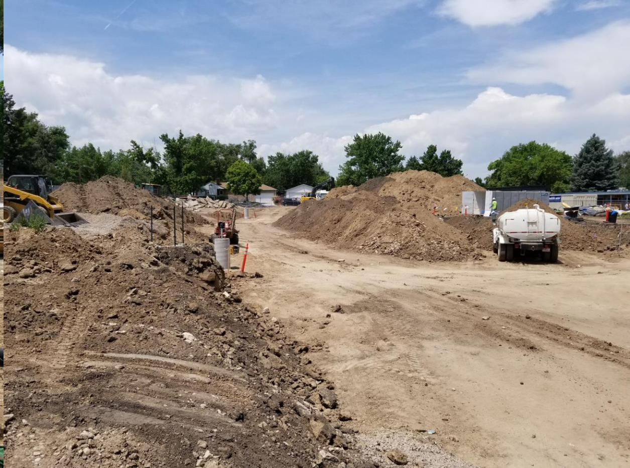
Southwest Corner of Property (Future Drive Aisle and Parking Lot) – Grading continues and installation of light poles.
