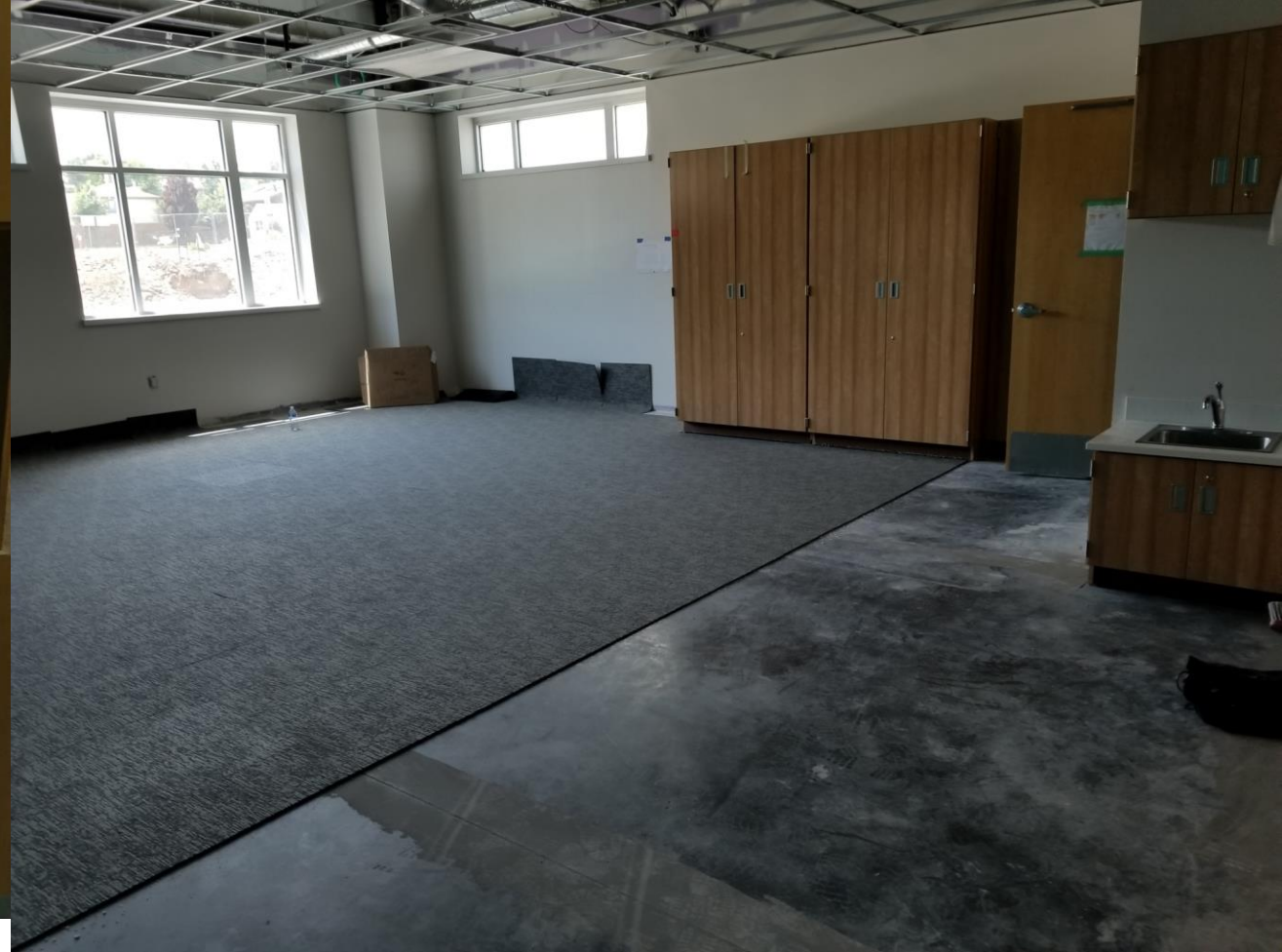
South Classroom Wing (L1) – Classroom; Floor being installed. Carpet install nearly complete.
