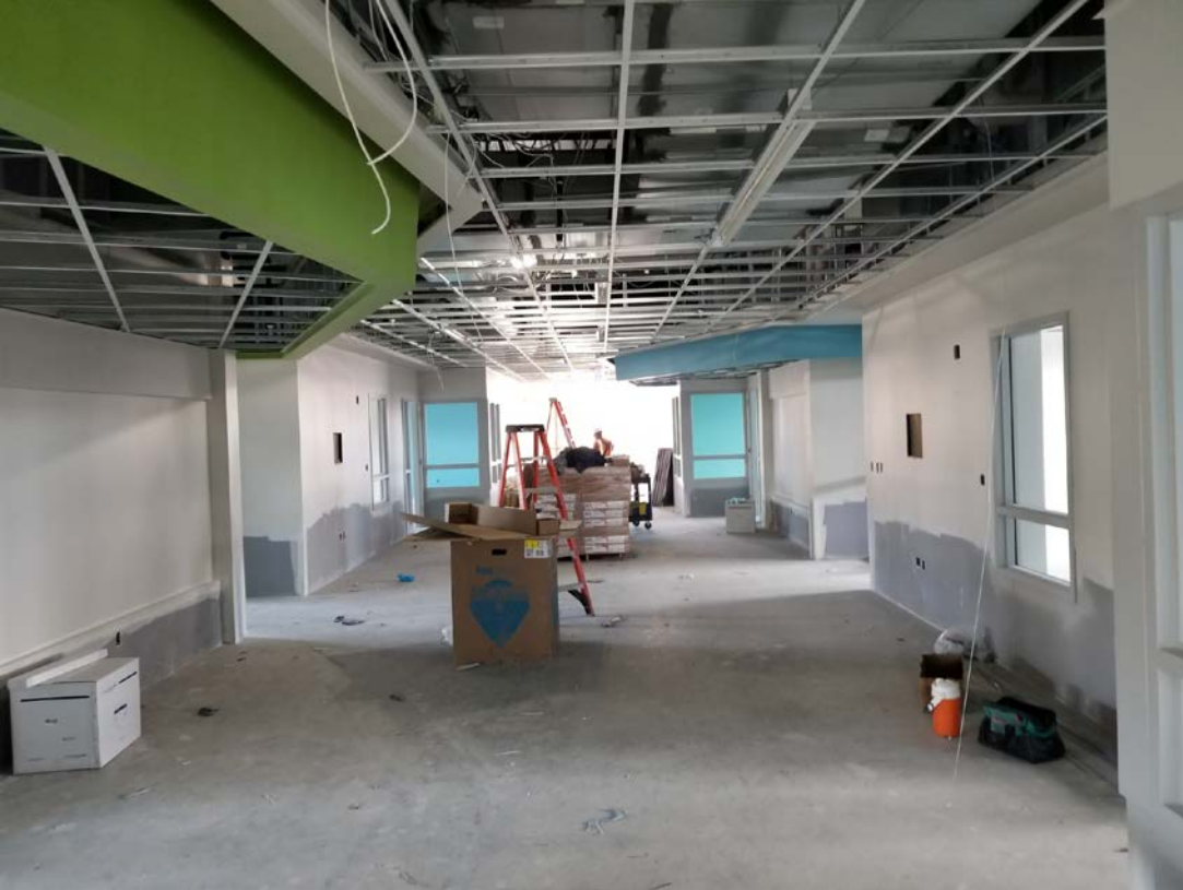
North Classroom Wing (upper level) – West Facing View; Ceiling install in progress and tile install next
