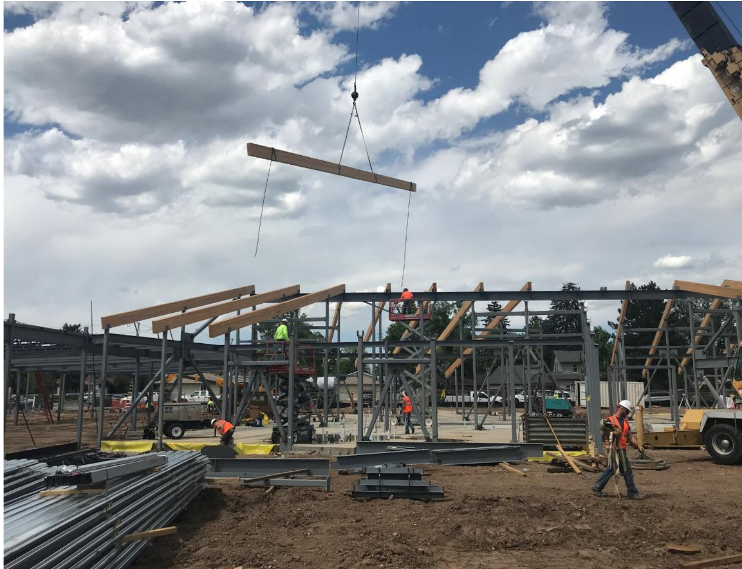
Glulam (glued laminated timber) beam installation.
