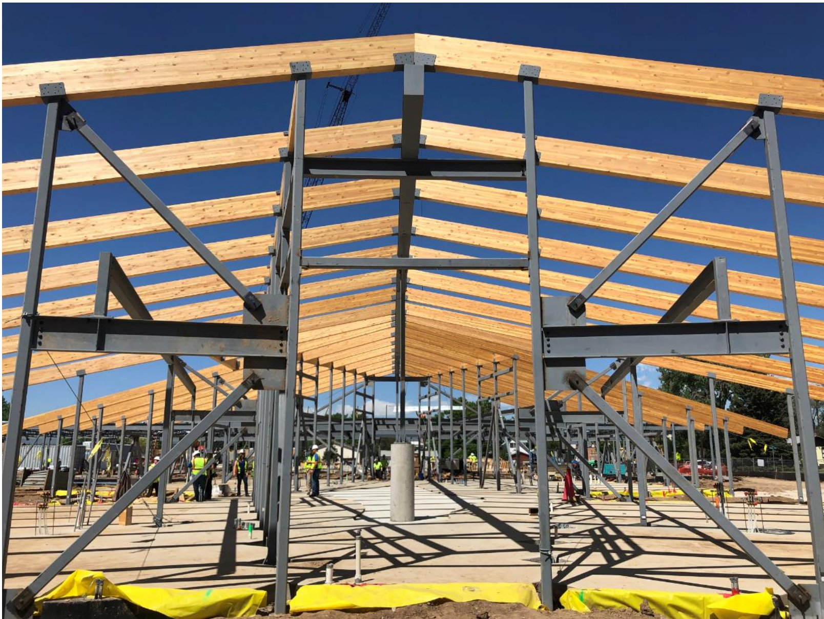
Looking West. Glulams installed on East wing.
