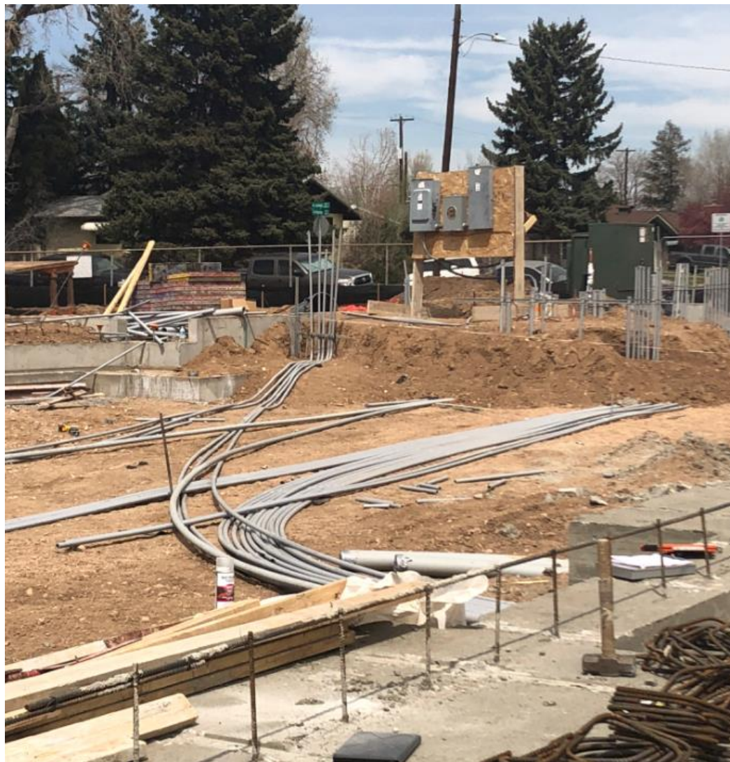
Underground conduit from electrical room.
