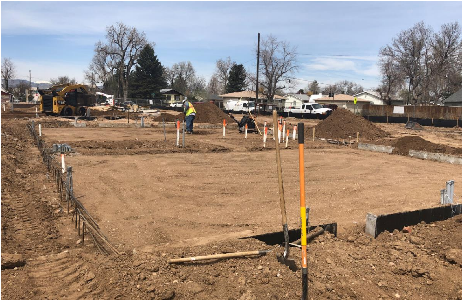
Preparing East wing for floor slab.
