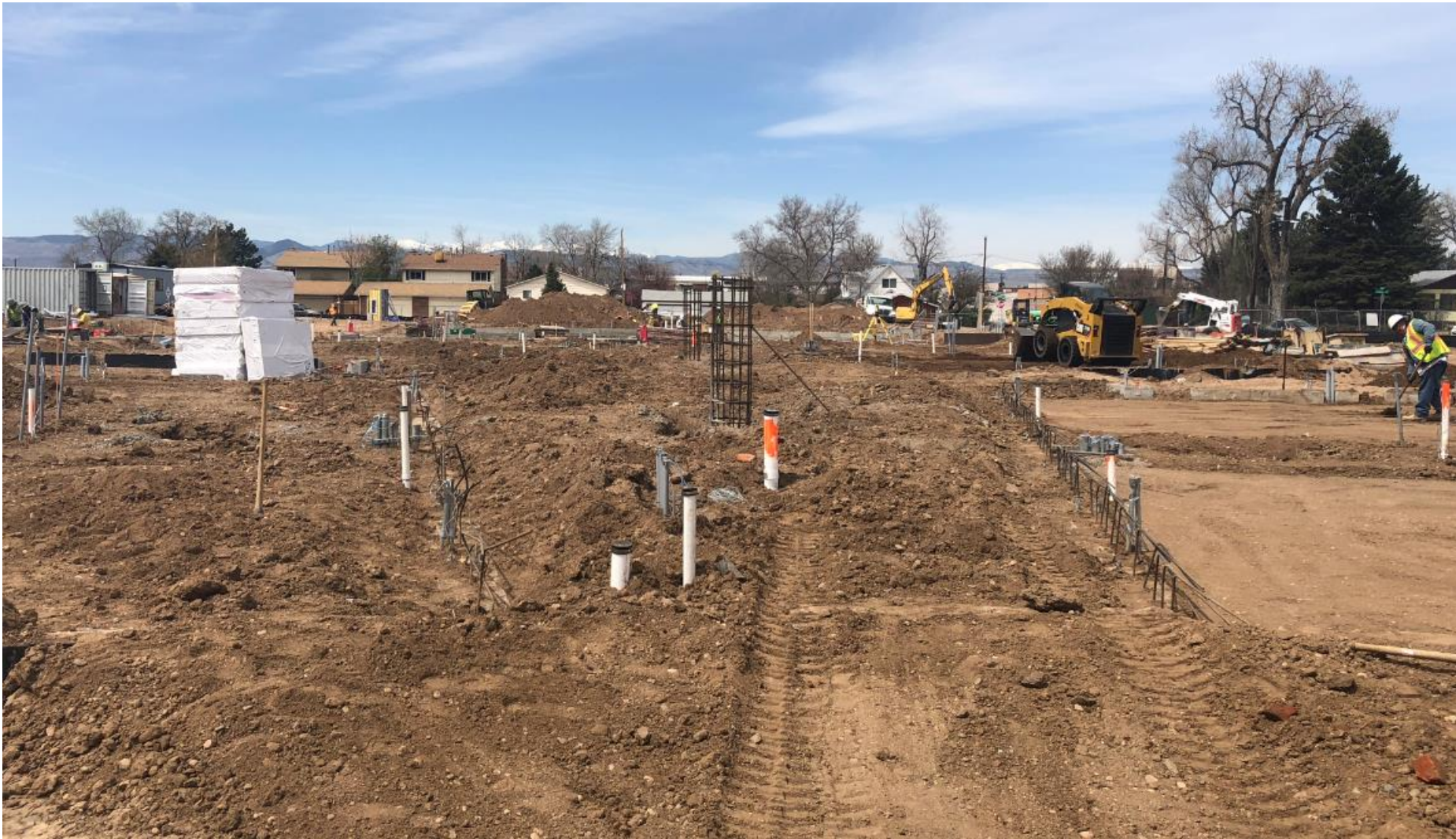
Looking West, rebar placed for columns.
