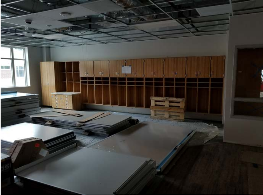
North Classroom Wing (L1) – Classroom; Ceiling tile to be installed.
