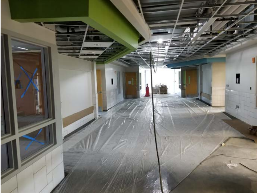
North Classroom (L1) – Ceiling tile to be installed.
