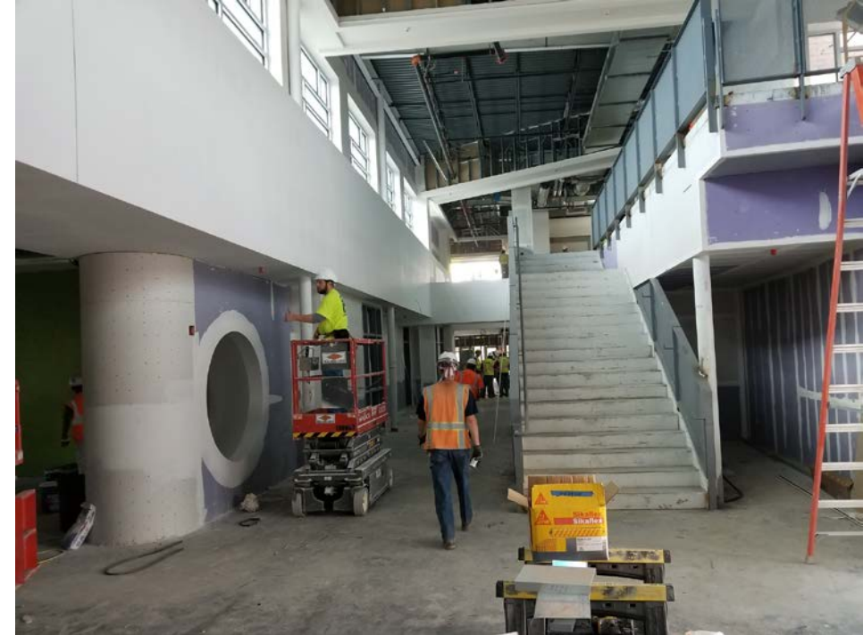
Grand Hall – South Facing; Ceiling being installed and painting in progress.
