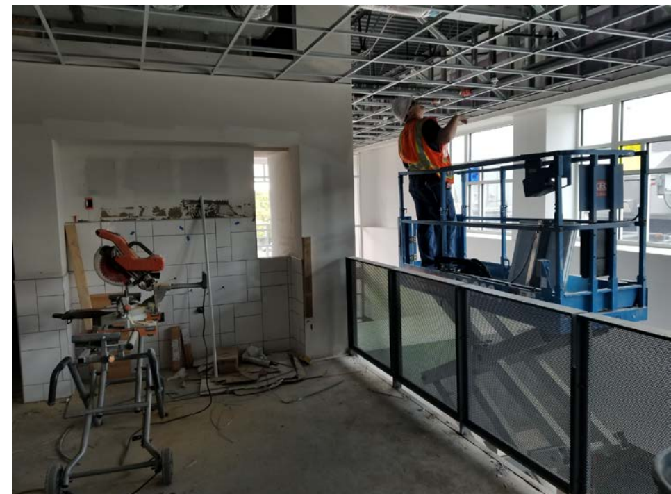
Grand Hall – South Facing View; Ceiling being installed.
